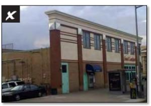
Non-continuous false front parapet without height changes
