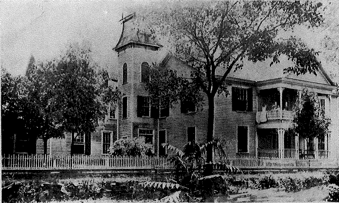
FRONT VIEW MAIN BUILDING
